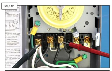
Test power hub power at the breaker/timeclock for 120 or 240vAC. IF correct, fix wiring/connections. IF not, resolve at breaker/timeclock.
