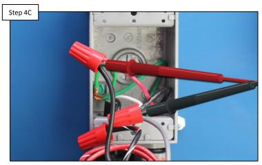
Verify line power to the Smart Relay between the grey & black (120vAC) or black & red/grey (240vAC). IF no/low voltage, correct at power source. IF correct, replace the Smart Relay (HLX485RELAY).
