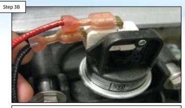
With power off, inspect the water pressure switch wiring for damage. IF damaged, replace the wire harness (pg. 20). IF OK, go to step 3C.
