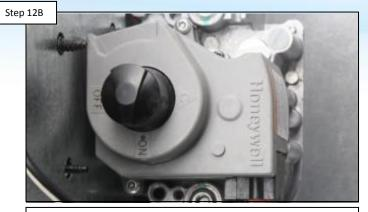
Verify that the gas valve, inside the heater, is in the "ON" position. IF correct, go to step 12C. IF NOT, rotate knob to ON position.
