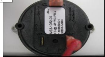
Disconnect wires from vent pressure switch and measure continuity between VPS terminals. IF open, replace the vent pressure switch (pg. 20). IF OK, go to 11I.
