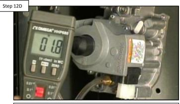
Ensure gas static, load, and manifold pressures are correct (See Page 16 & 17). IF OK, go to Step 12E. IF NOT, go to Step 12F.
