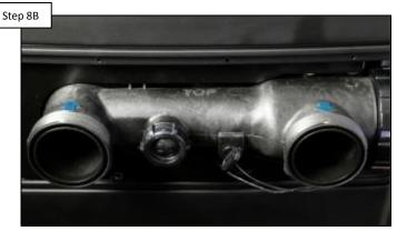
Verify the water inlet & outlet are not reversed; reversing these will often cause frequent occurrences of the "HS" error code. Follow the steps outlined in 8A. IF the thermistor checks-out, replace the ICB (pg. 20).
