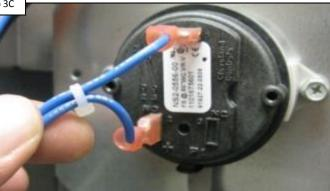
With power off, inspect the blower vacuum switch wiring for damage. IF damaged, replace the wire harness (pg. 20). IF OK, go to step 3D.
