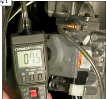
The static & load values should be within the levels listed on the data plate, example on Page 17. Measure the outlet manifold pressure (valve on / energized), as shown below.
