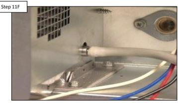
Applies To Indoor Installations ONLY: Inspect the vent pressure switch tube connections. IF OK, go to 11G. IF NOT, repair/replace tubing (pg. 20).
