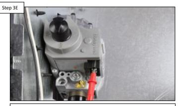
With power off, measure resistance, comparing each terminal to ground. IF any terminal shows continuity, replace the gas valve (pg. 20). IF OK, go to step 3F. **ICB** wiring
