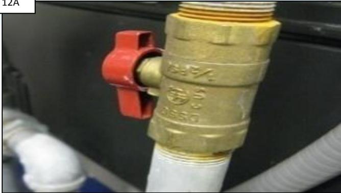
IF "Ignition Failure", Ensure main gas supply is in the ON position. IF ON, go to step 12B. IF NOT, open gas supply.
