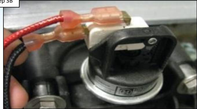
With power off, inspect the water pressure switch wiring for damage. IF damaged, replace the wire harness (pg. 20). IF OK, go to step 3C.
