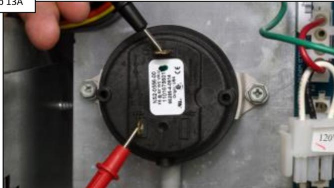
Isolate the blower vacuum switch. Measure continuity between switch terminals. IF continuity exist, replace switch (pg. 20). IF OK, go to 13B.
