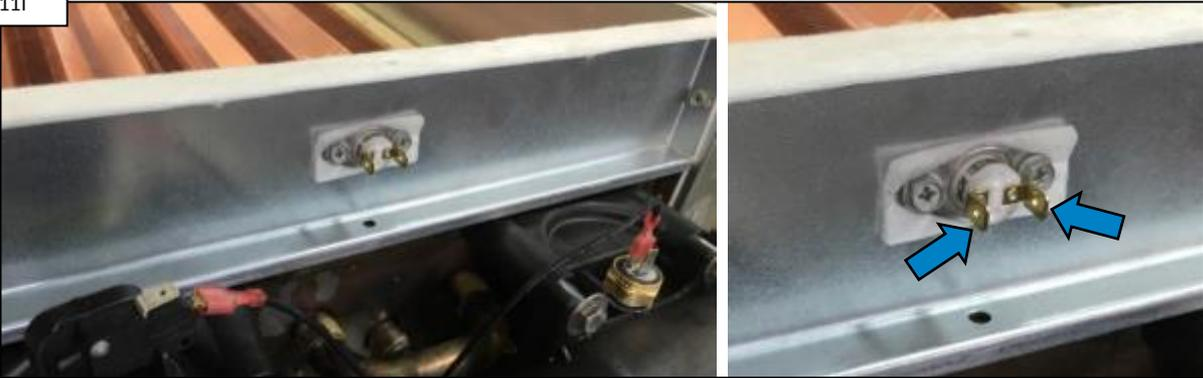
**Test continuity across the exhaust gas limit switch. IF open, replace switch ([pg. 20](#)). IF switch does not exist AND problem still persists, contact support: (908) 355-7995**
