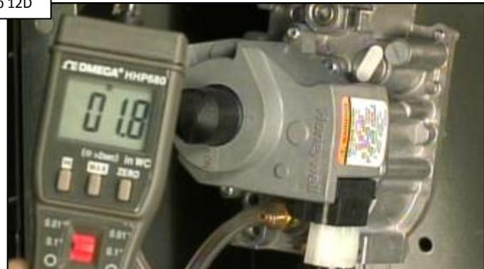
Ensure gas static, load, and manifold pressures are correct ([See Page 16 & 17](#)). IF OK, go to Step 12E. IF NOT, go to Step 12F.
