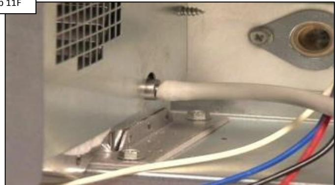
Applies To Indoor Installations ONLY: Inspect the vent pressure switch tube connections. IF OK, go to 11G. IF NOT, repair/replace tubing (pg. 20).
