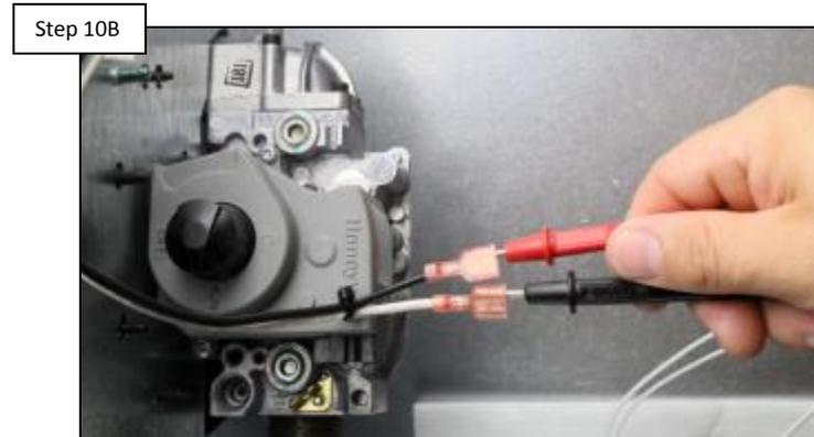
Press the mode button to toggle the heater and call for heat. IF 24VAC is still present at gas valve AND manifold pressure is not present, gas valve is defective and needs to be replaced. Otherwise, replace the ICB (pg. 20).
