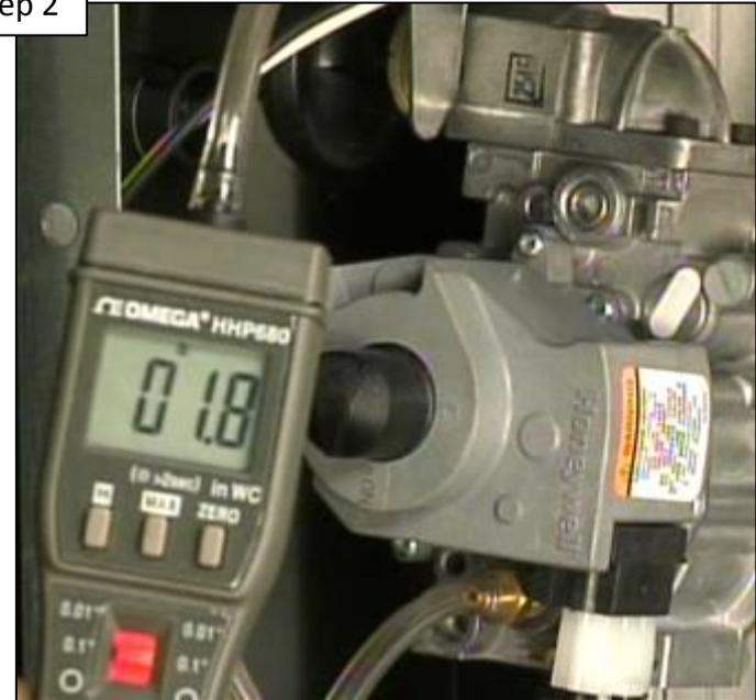
Manifold reading should be between 1.8" - 2.0" w.c for natural Gas or 6.8" - 7.0" w.c for propane.
