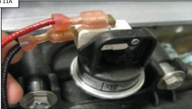
Inspect the water pressure switch wiring, ensuring wire harness terminals are securely fastened. IF damaged, replace wire harness ([pg. 20](#)). IF secure and free of damage, go to step 11B.
