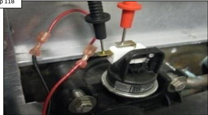
Remove wires from water pressure switch & measure continuity across terminals (while pump is running). IF open, replace water pressure switch. IF OK, go to Step 11C.
