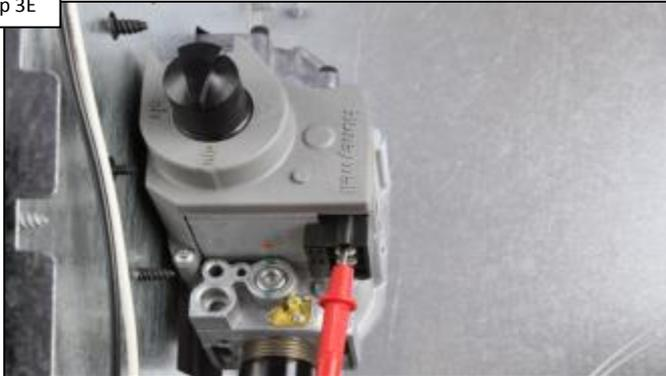
With power off, measure resistance, comparing each terminal to ground. IF any terminal shows continuity, replace the gas valve (pg. 20). IF OK, go to step 3F.
