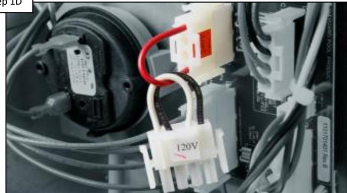
Verify selector plug matches incoming line power. IF it does not, power OFF & correct. IF OK, go to 1E.
