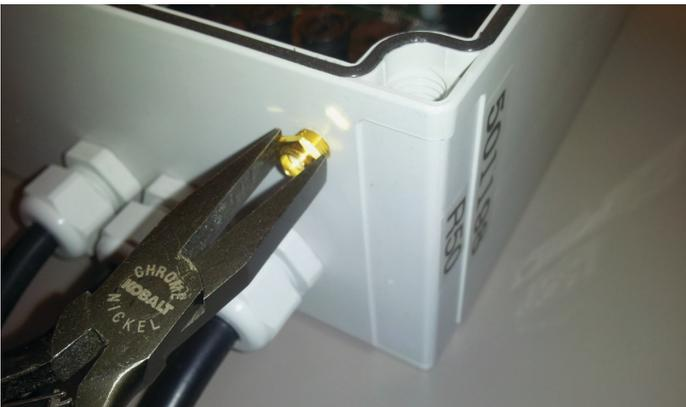
5) Remove old antenna cable from housing.
